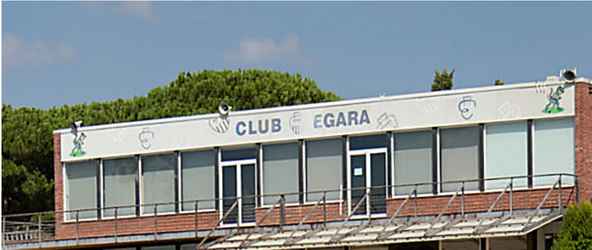
Figure 32. Wall 11 Social Building
