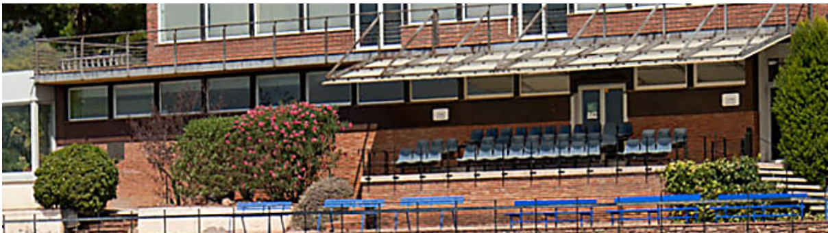
Figure 31. Wall 10 Social Building
