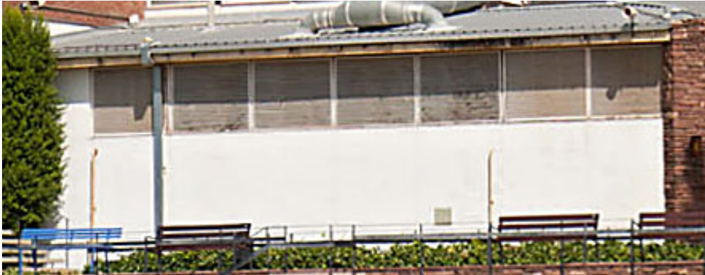
Figure 30. Wall 9 Social Building
