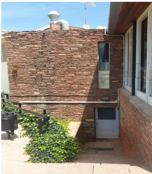
Figure 28. Wall 7 Social Building
