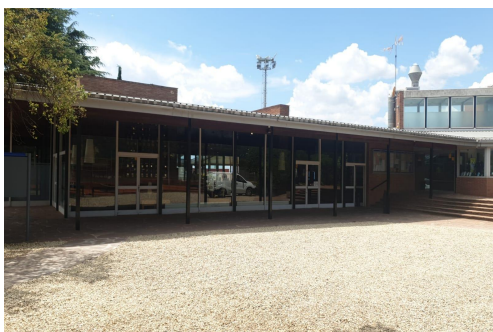
Figure 24. Wall 3 Social Building
