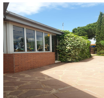
Figure 25. Wall 4 Social Building
