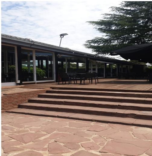
Figure 26. Wall 5 Social Building
