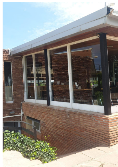
Figure 29. Wall 8 Social Building
