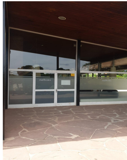
Figure 27. Wall 6 Social Building
