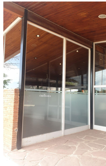
Figure 23. Wall 2 Social Building
