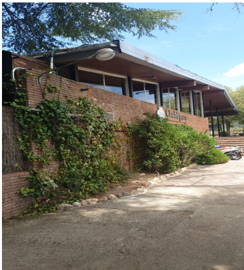
Figure 22. Wall 1 Social Building
