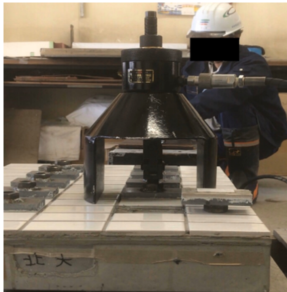
Figure 3.11: Removing the tile.
