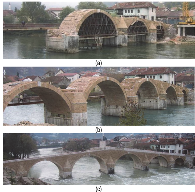
Figure 2 KB: a) bridge Arch Completed on a Pier; b) completed Bridge Arches; c) general view [40]
