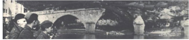
Figure 1 The collapse of the KB during World War II (1945) [40]
