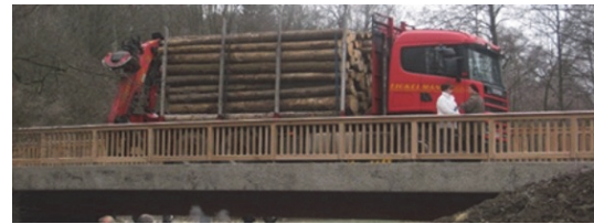
Figure 1 Pioneer of TCC bridges in Germany [34]
