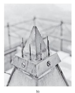
**Fig. 10.** Toping of the Washington Monument: a) illustration of placing the cap [83], b) cast Al cap with lightning-rods [84]
