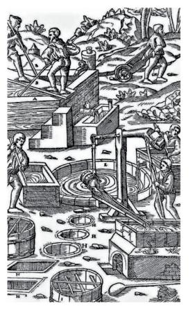
A – tanks, B – stirring poles, C – plug, D – trough, E – reservoir, F – launder, G – lead cauldron, H – wooden tubs sunk into the earth, I – vats in which twigs are fixed
