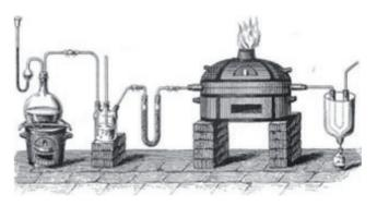
Fig. 8. Ørsted's apparatus for synthesis of dry aluminum chloride [76]
