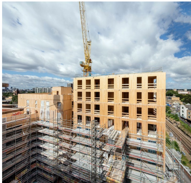
Figure 8: Dalston works during construction, London (walsh, 2018)
