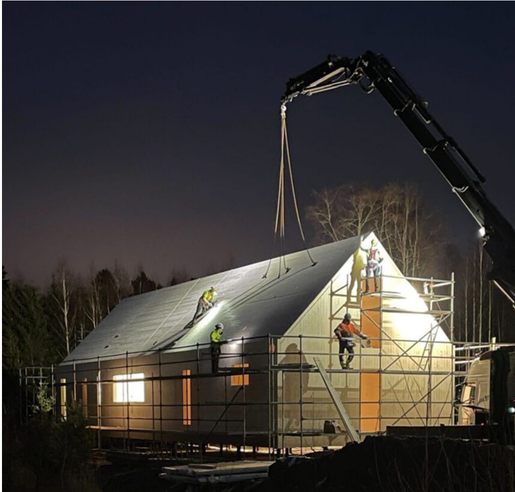
Figure 9: CLT dwelling by Asumma in construction (Mela, 2013)
