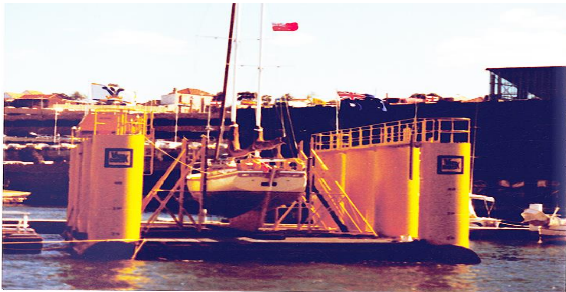
Figure 13 Vick Dock floating dock (Source: Alison Cole)
