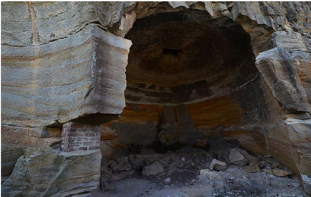
Figure 06 Cockatoo Island convict wheat silo. Between 1839 and 1841 twenty were quarried. (Source: Wikimedia)
