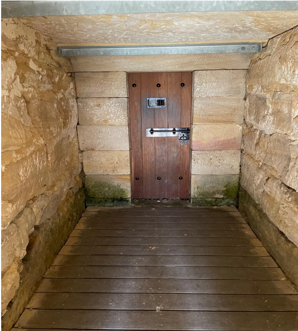
Figure 02 Restored solitary confinement cells, internal (Source: Alison Cole)
