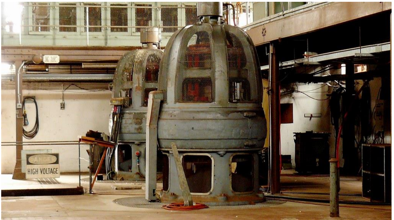
Figure 05 Powerhouse on Cockatoo Island (Source: flickr)
