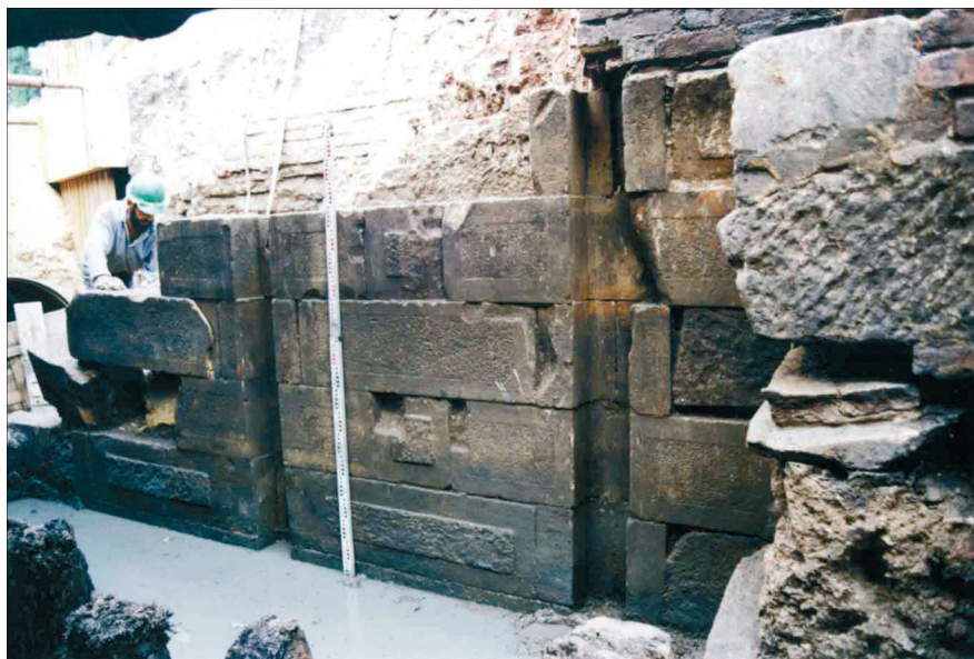
Fig. 16. Wrocław, Ketzerkunst water house, interior of building above moat, visible inlets for fixing wooden structures (photo by P. Konczewski)
