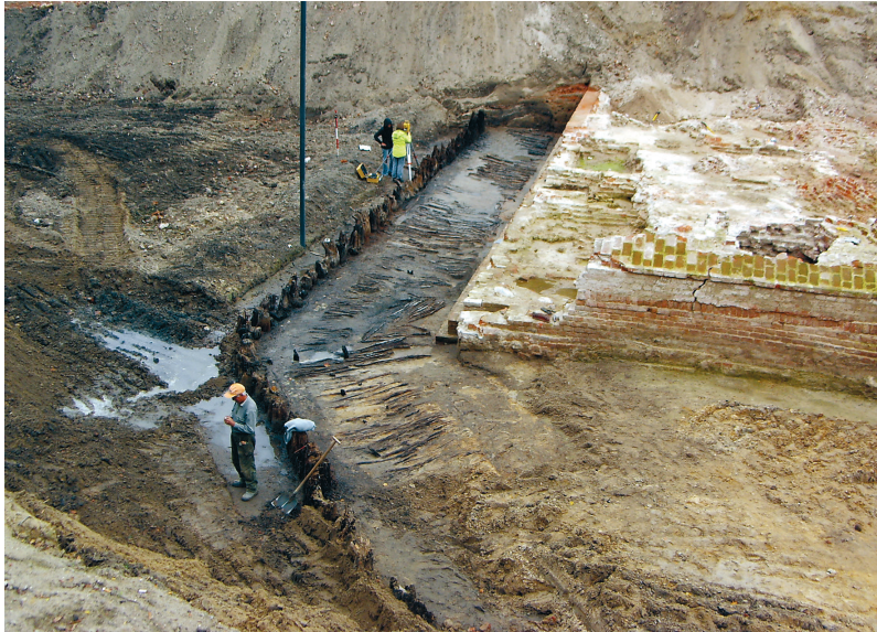
Fig. 8. Krupniczy Bastion during excavation works. View of left flank, part of the face and projecting outwards, strengthened with posts, fascine platform (after Konczewski, Mruczek et al. 2010)
