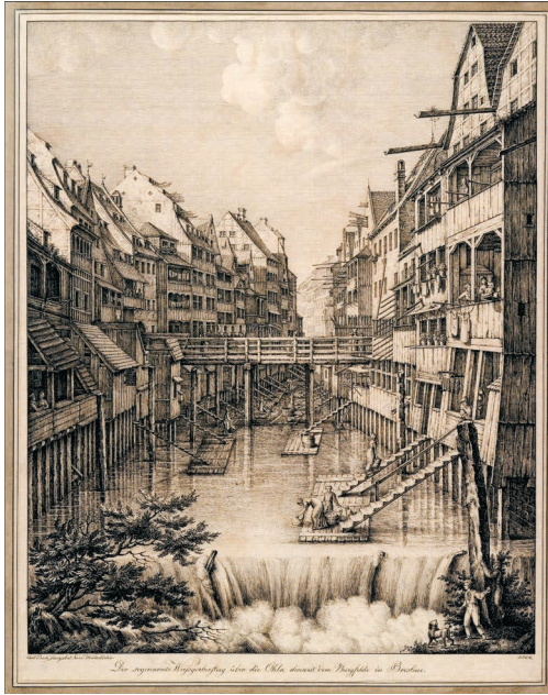
Fig. 19. Wrocław, Białoskórnicza Street. Inner moat in 1826, drawing by Heinrich Mützel (after Ikonografia Wrocławia 2008)
