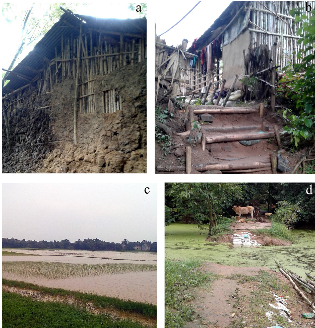
Fig. 3. Severity of flood, a. and b. Dilapidated kutcha (muddy/thatched) houses due to flood in Hijal, Murshidabad c. Inundated land in Hijal d. Breaching of the pakka (concrete) road by flood (Source: Field photographs 2018)
