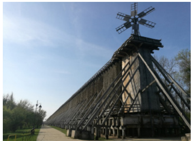
Fig. 1. Brine graduation towers No. 1 in Ciechocinek Source: photo M. Kejna
