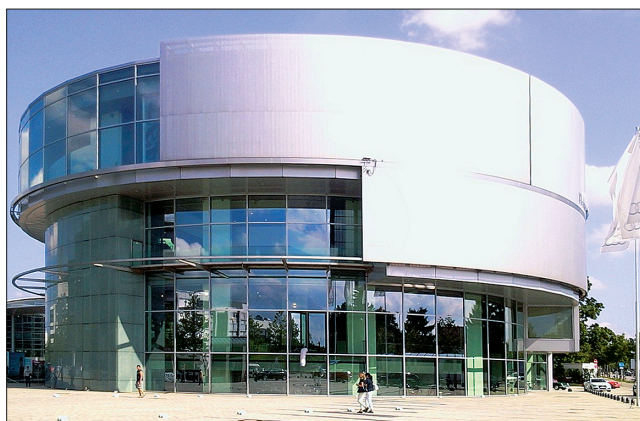
Fig. 3. The Museum Mobile building
