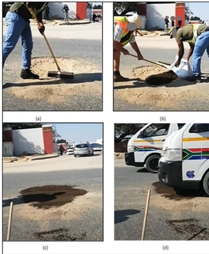
Figure 6: Pothole repair using a MC-NME mix, (a) Cleaning of the pothole and “painting” of pothole with anionic NME liquid, (b) filling pothole with a water-resistant anionic NME mix, (c) pothole filled and partially compacted by hand, and (d) vehicles driving over filled pothole
