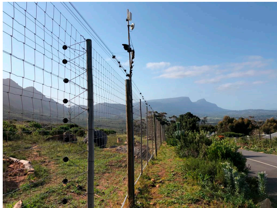
Figure 1. The baboon-proof electric fence in the suburb of Zwaanswyk in Cape Town. Photo © Jessica Burnette, 2020.
