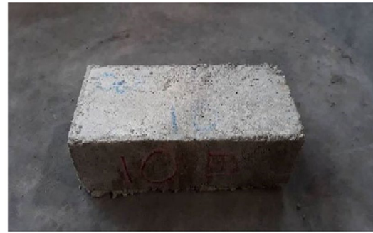
Slight - When thin deposit of salts is covered over exposed area of the concrete is less than 10%.
