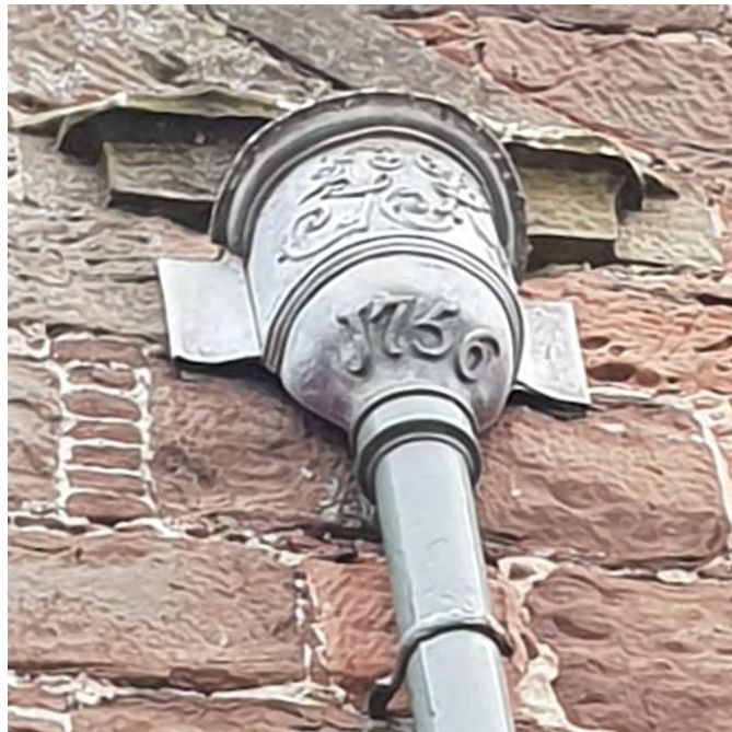
Figure 2.12. Royal cipher and date on hopper head of downpipe, Fort George, Ardersier. Author photograph.
