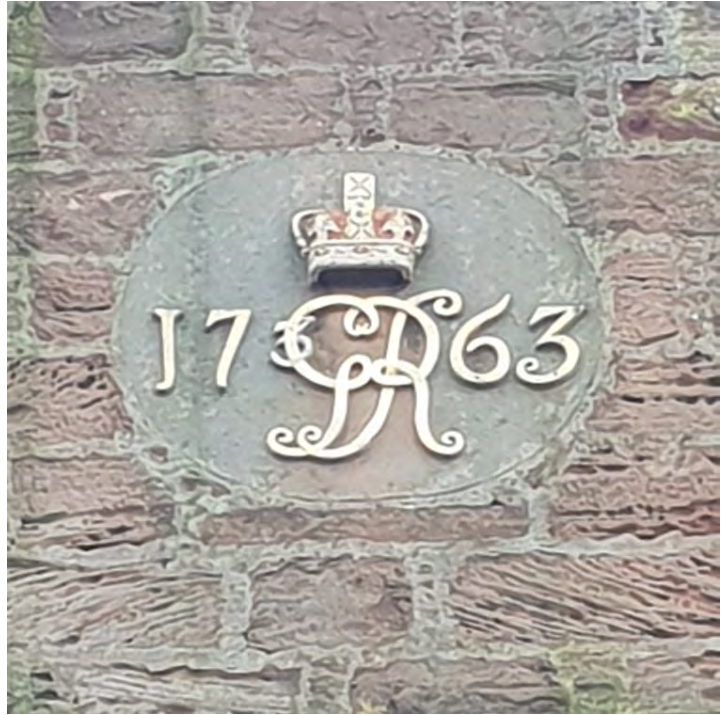
Figure 2.11. Royal cipher on barracks pediment, Fort George, Ardersier. Author photograph.
