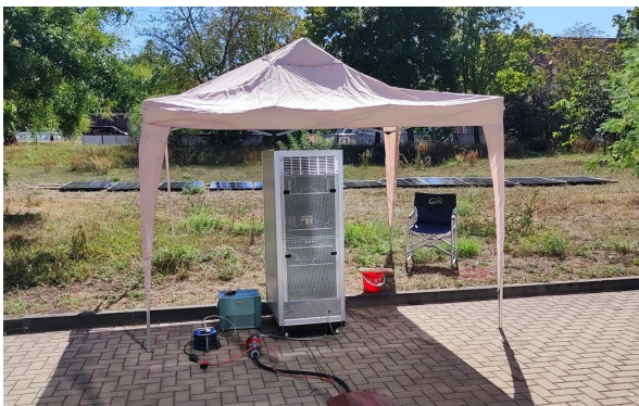
Fig. 3. Case study 1. System under test in the outdoor test site. The photo shows the DC-AC inverter with 12 PV panels behind it.
