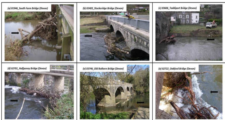
Fig. 3 Images of wood accumulation at some of the study bridges. The arrows indicate the direction of river flow. Source: Devon County Council (2018)
