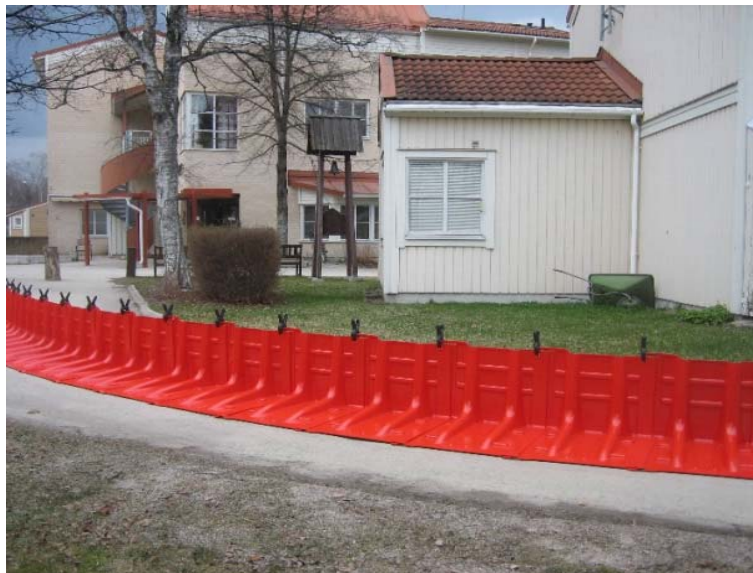
(B) Temporary Flood barrier
