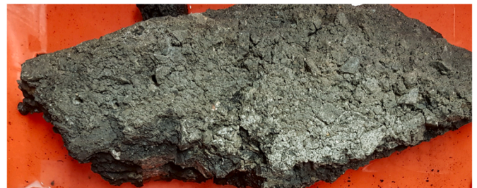
Fig. 10. Application example: Piece of asphalt with holes and naturally formed fissures.
