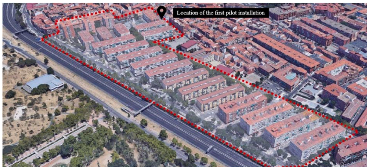
Fig. 10. Urban Regeneration Area “La Alhóndiga” with the location of the first prototype installed [56].
