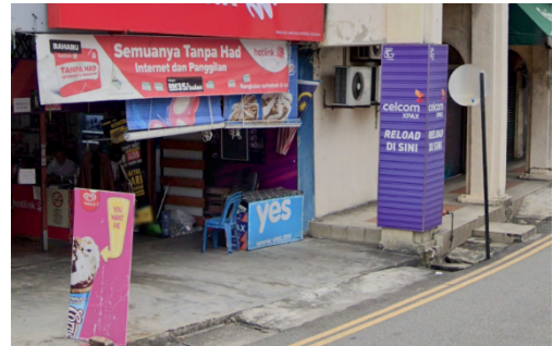
Figure 1.2 Lack of drop curb
