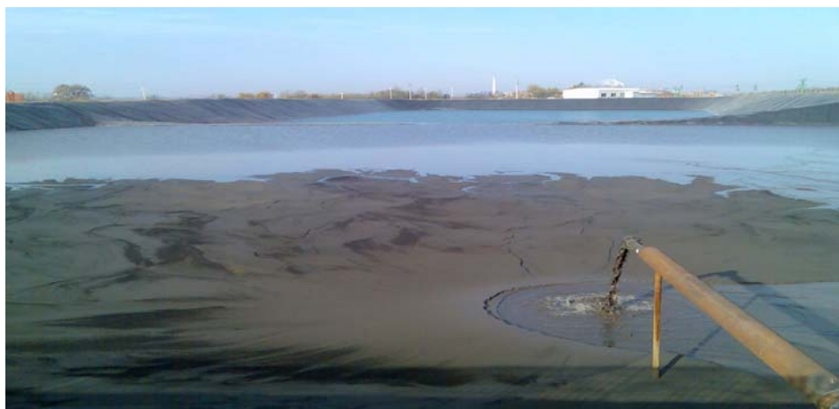
Figure 2. Ash and slag settling basin in Medoševac – primary settling in the small settling basin.
