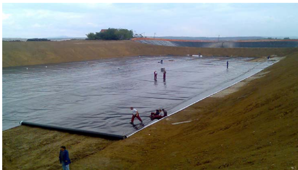
Figure 1. Setting up of the geomembrane in the large settling basin
