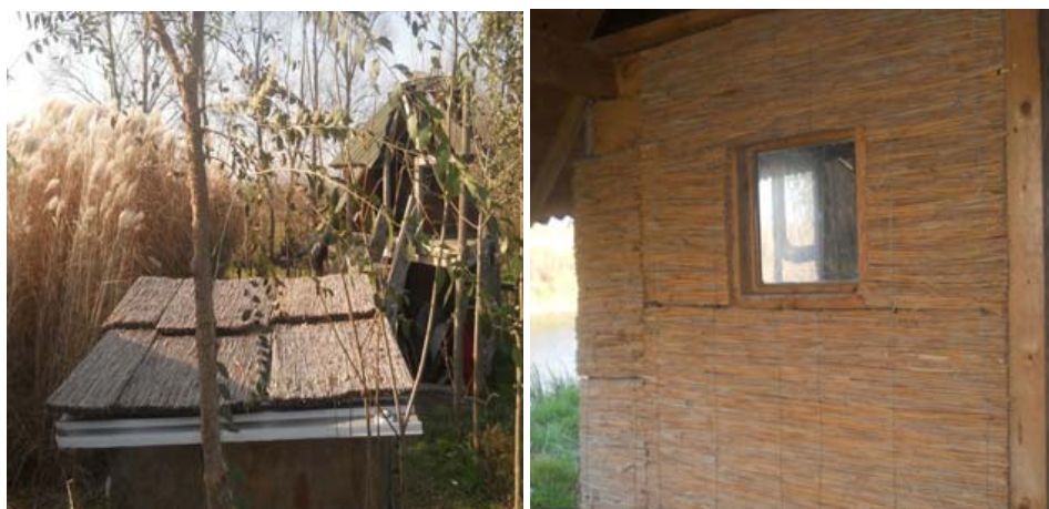
Figure 2. Cottage built with Miscanthus Giganteus panels
