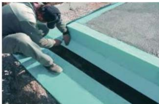
Figure 6. Placing of XPS isolation
