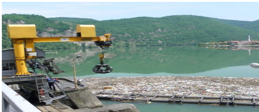
Figure 5. The largest pieces of floating debris are taken out by grapples (the example from 'Zvornik hydropower plant')
