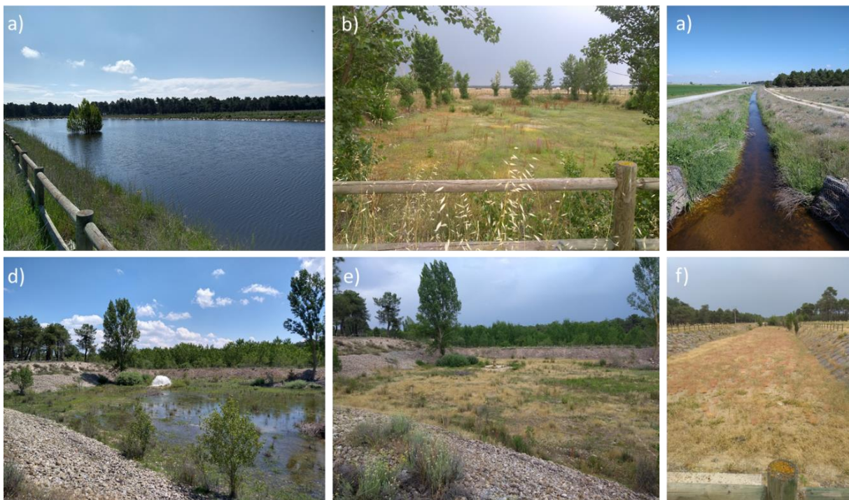
Figure 11. Some of the infrastructure of the Los Arenales MAR systems: a) Santiuste infiltration basin during a recharge cycle; b) relatively small infiltration basin in the area of El Carracillo; c) infiltration channel connected to the Santiuste infiltration basin; d) La Laguna del Señor infiltration basin during a recharge cycle (El Carracillo area); e) La Laguna del Señor infiltration basin during a dry cycle; f) large infiltration basin in El Carracillo area. The pictures were taken between 2020 and 2022.
