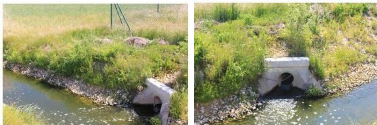
Figure 71. Purified water from the Santiuste village's waste water treatment plant (by lagooning) is poured into the MAR channel. Los Arenales Aquifer, Spain.
