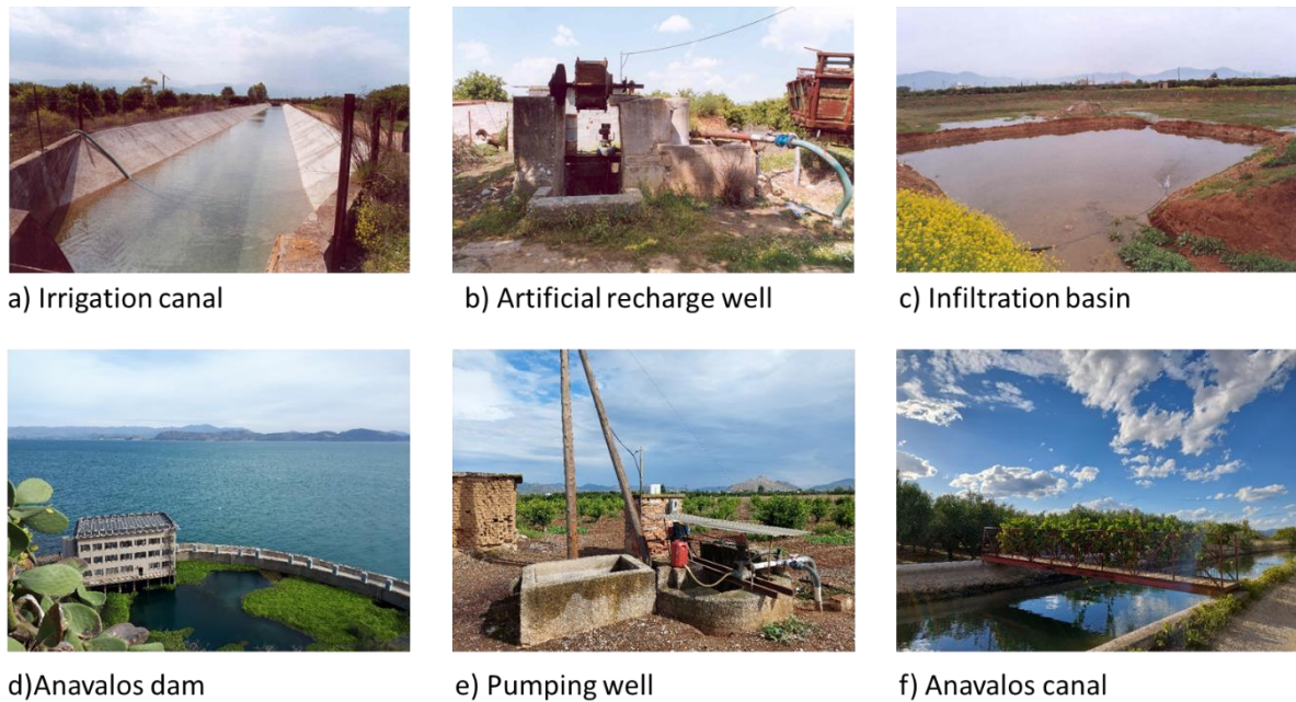
Figure 48. The infrastructure system of water resources management (MAR and irrigation) in the Argolis field. Water is transported from the Anavalos dam through the Anavalos canal.
