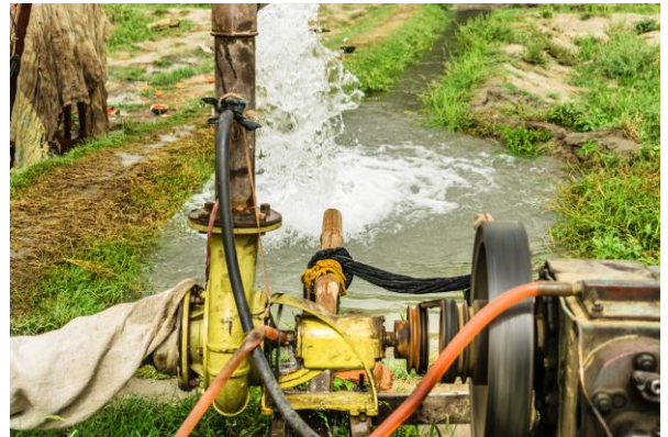
FIGURE 6: GROUNDWATER PUMPED BY A DIESEL ENGINE IN PAKISTAN. (IMAGE: ZMS)
