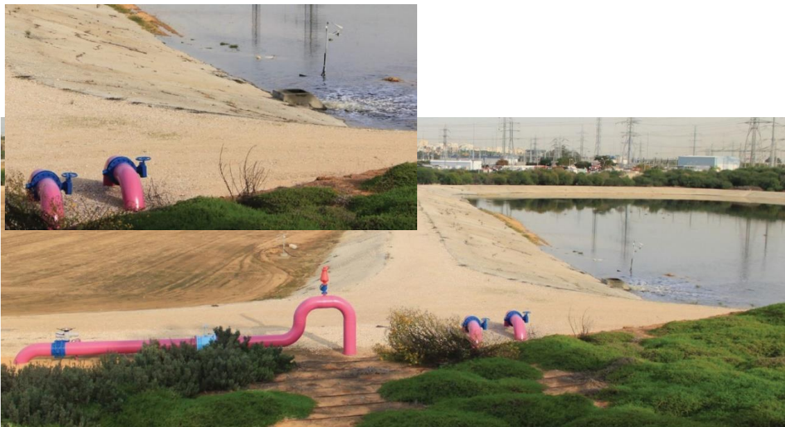
Figure 11. MAR regulated system in Shafdan, Israel. Sensors inside the infiltration basins allow the water quality monitoring in real time, in order to attain the standards of quality. From Fernández Escalante et al. (2020).
