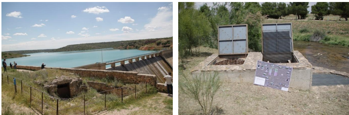
Figure 31. The Guadiana MAR site: (a) Peñarroya dam heading the MAR canal), and (b) MAR well used to recharge river water into the mudstone aquifer. Photos of the authors.
