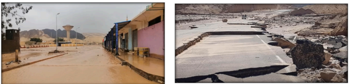
Fig. 2. Heavy Rain Abou Zenima City on the 12 th of March 2020.
