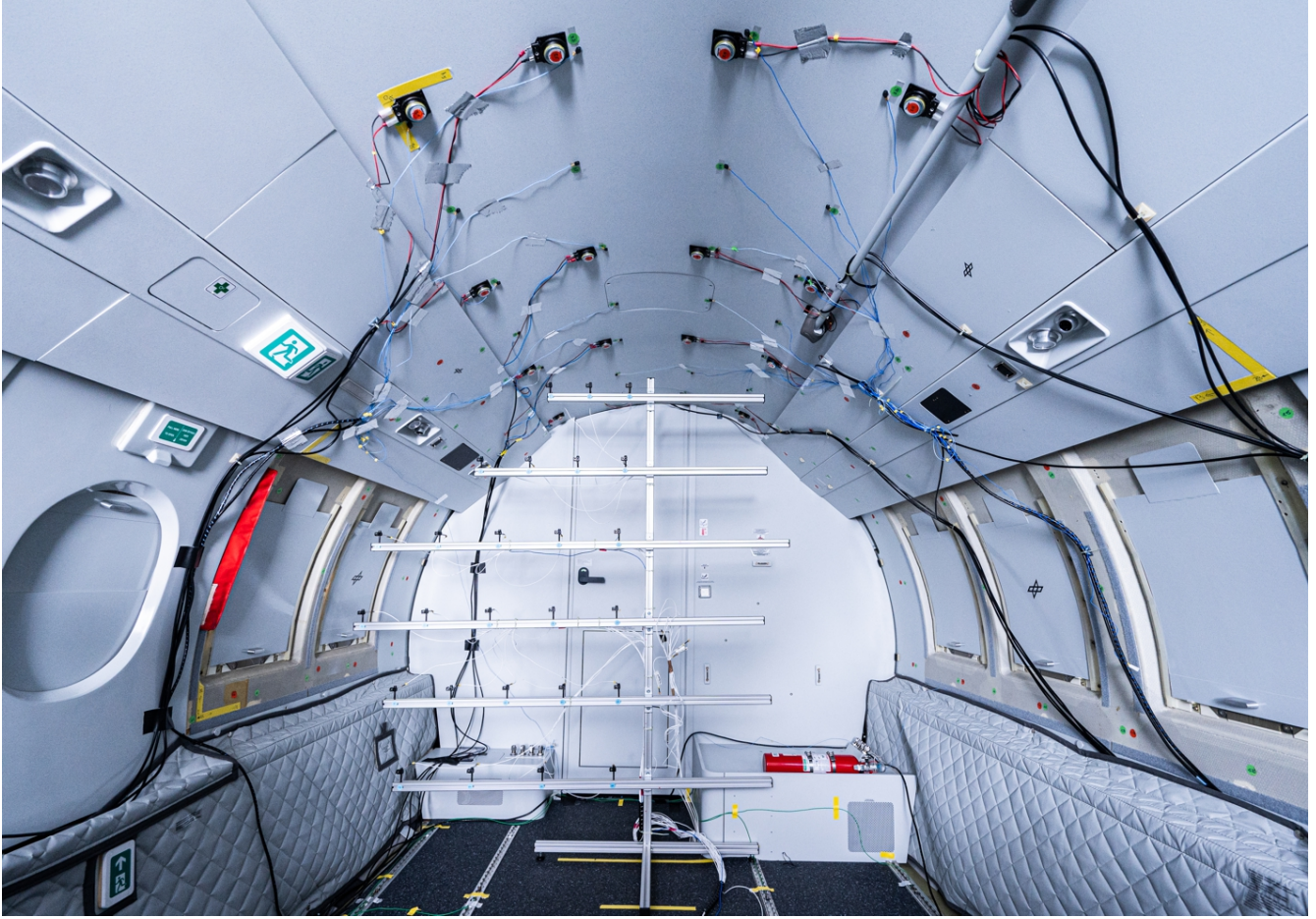
Figure 3: Photo of test setup in aft of iSTAR cabin. 16 inertial exciters on the ceiling panel marked with red dots and 26 microphones on a movable stand in configuration 11 (C11) of Fig.2.
