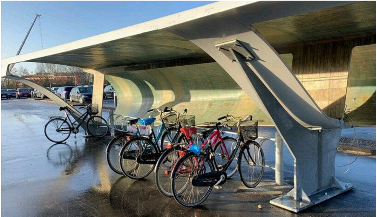
Figure 9. Wind turbine blades being used as a bike shed in Aalborg, Denmark (designboom, 2021).
