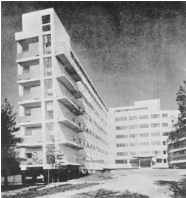
Figure 6.8. Paimio Sanitarium. William H. Jordy, "PSFS: Its Development and Its Significance in Modern Architecture," Journal of the Society of Architectural Historians 21, no. 2 (May 1962):82
