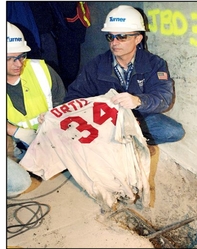
Figure 2.5. Red Sox jersey recently freed from the concrete of Yankee Stadium. AP Photo/Frances Roberts.
