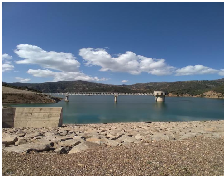
Figure 3. Kef Eddir dam in the wilaya of Tipaza
