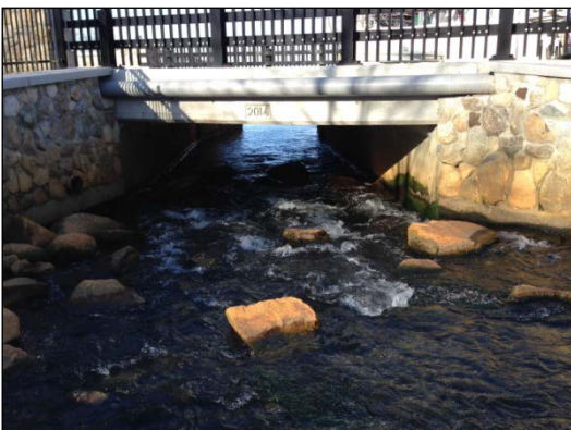
Water Street tidal rock ramp, Town Brook, Plymouth, MA
