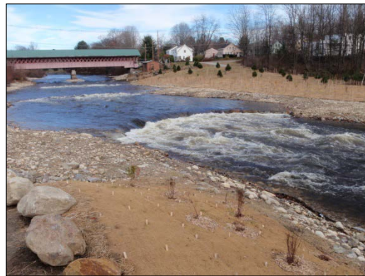
Homestead dam removal and NLF cross-vanes, Ashuelot River, West Swanzey, NH
