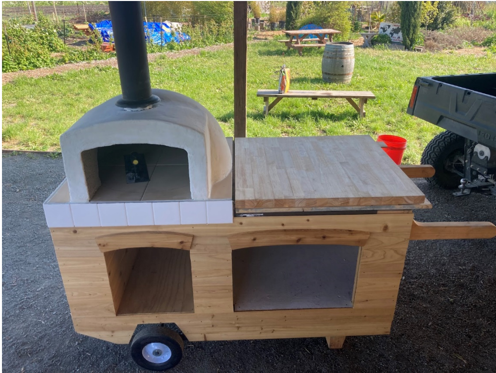
Figure 11: Arches Finished/ Tile Installed and Grouted/ Grout Layer Applied to Dome
