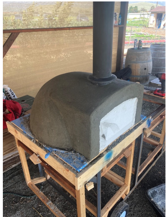
Figure 9: Stucco Layer Finished
