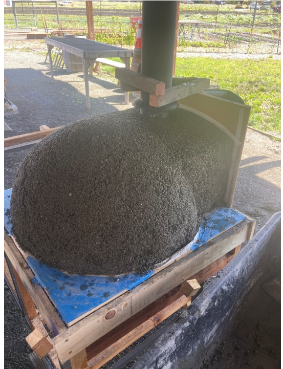
Figure 7: Perlite Cement Cast
