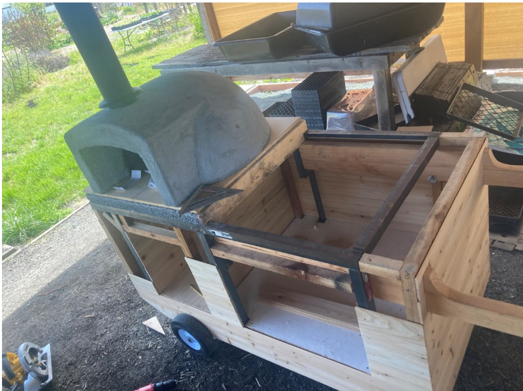
Figure 10: Installation of Cedar Siding
