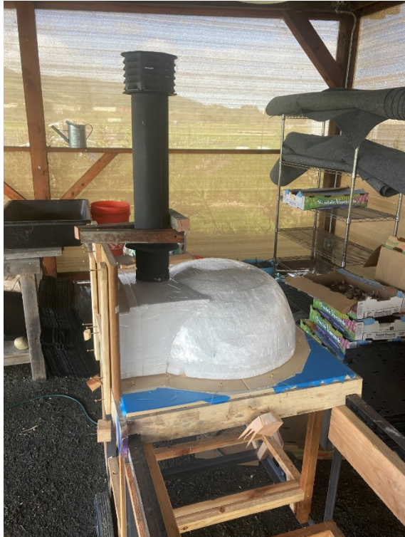
Figure 6: Ready for Dome Cast
