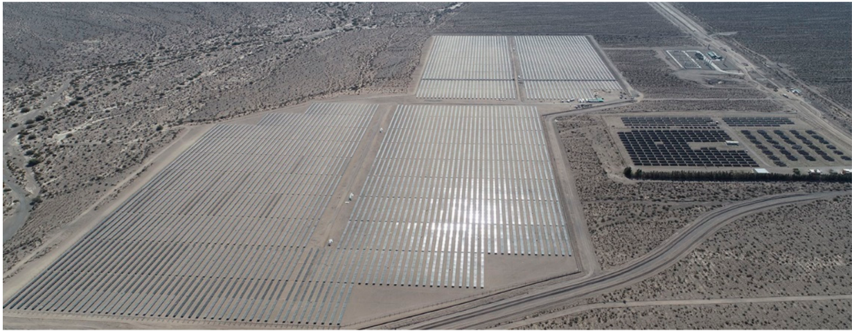
Figure 4. A view of Ullum IV, a 16 MWp photovoltaic plant located in the desertic province of San Juan, which went operative in 2019. Also shown is the San Juan I PV technology testing plant (far right, center). Photograph courtesy of Estrada.
