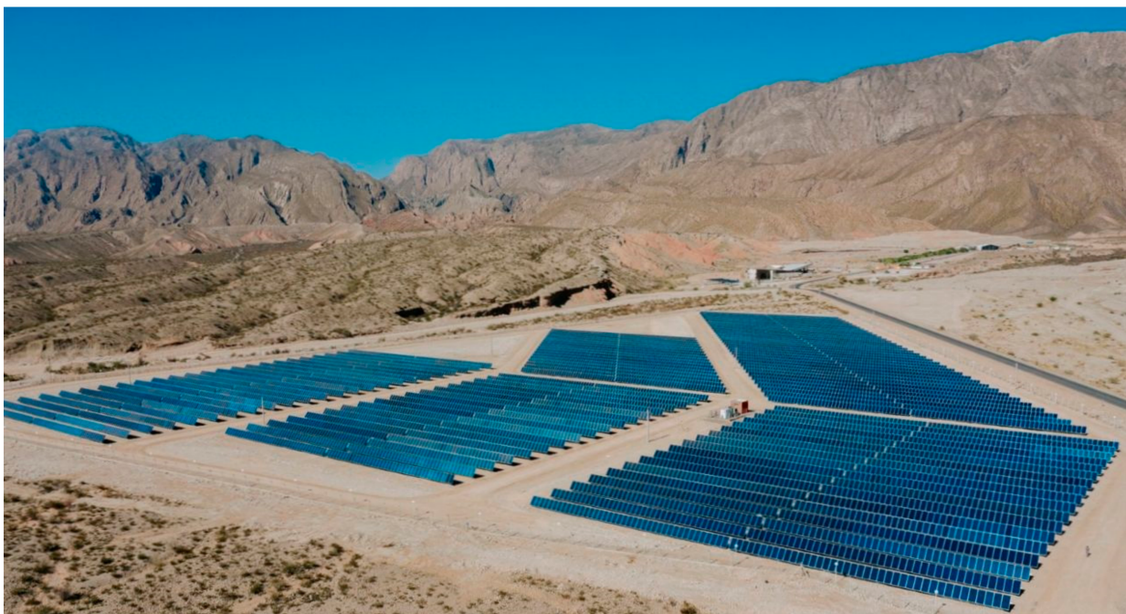
Figure 5. Anchipurac is a small-sized 3 MWp PV solar plant provided by single-axis tracking, located in Argentina’s west-central province of San Juan. Photograph courtesy of Estrada.
