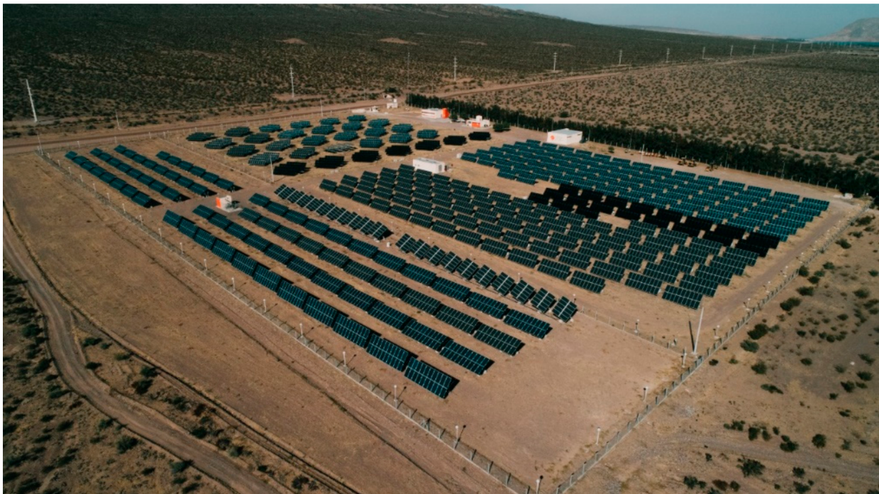
Figure 7. Solar San Juan I pilot solar plant, a 1.2 MW test facility using different module and mounting technologies, including fixed and single axis orientation for crystalline, multicrystalline and amorphous silicon modules. Photograph courtesy of Estrada.
