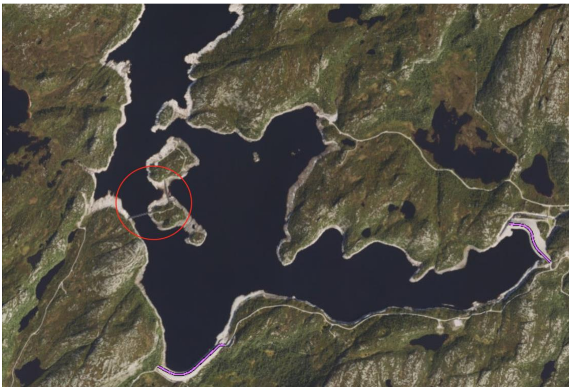
Figure 2: Upstream reservoir from Skjerka power station. The new dams are shown with purple, and the old dams separating Nåvatn and Skjerkevatnet are marked with a red circle (NVE Atlas).
