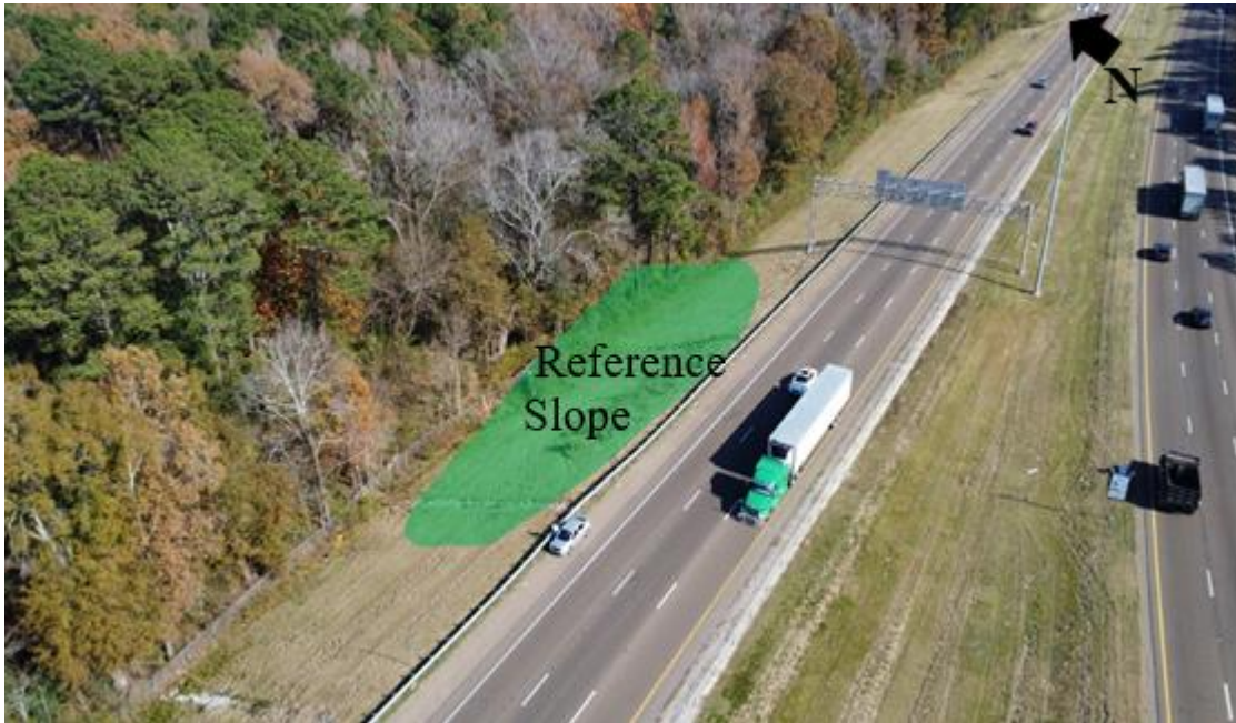
Figure 3.33 Location of I-Slope 4
