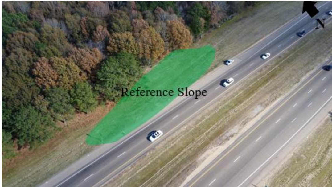
Figure 3.50 Location of I-Slope 6
