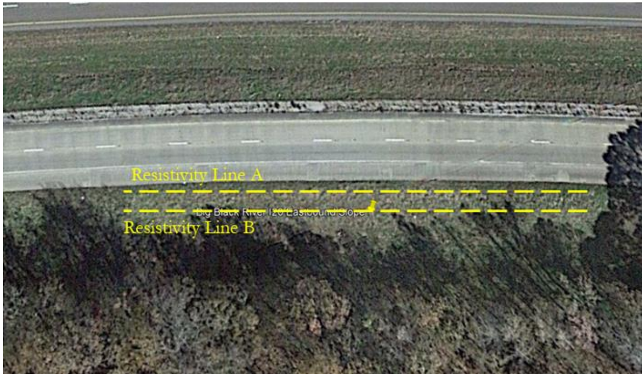
Figure 4.94 ERI Test Lines in Failed Slope 12
