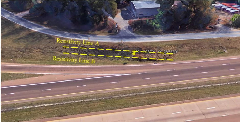
Figure 4.112 Location of ERI Test Lines in Failed Slope 18
