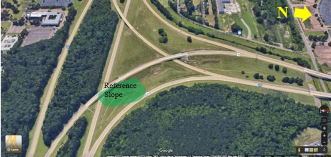
Figure 3.60 Location of I-Slope 7
