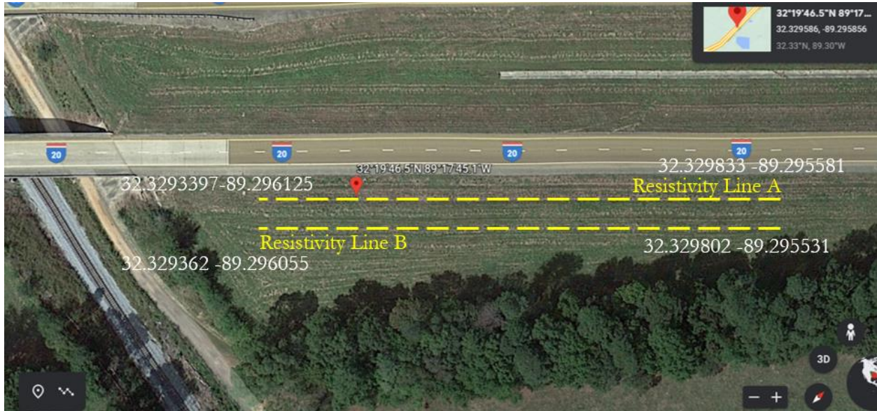
Figure 4.52 Location of Failed Slope 2
