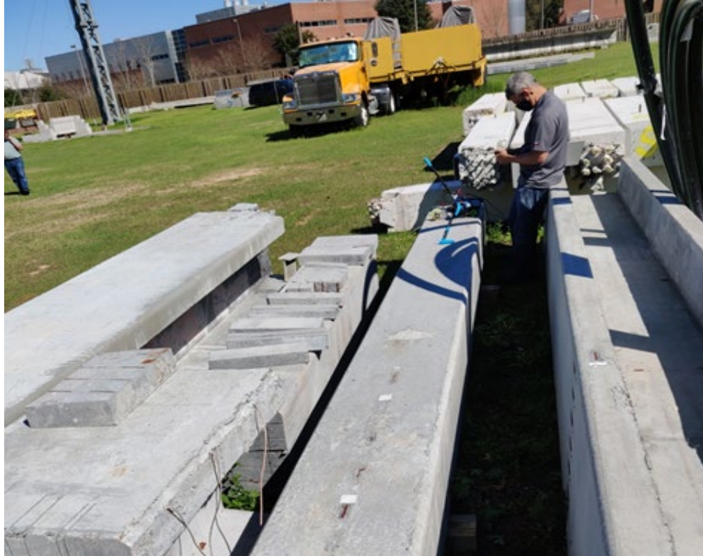
Figure 227: Square pile during scanning
