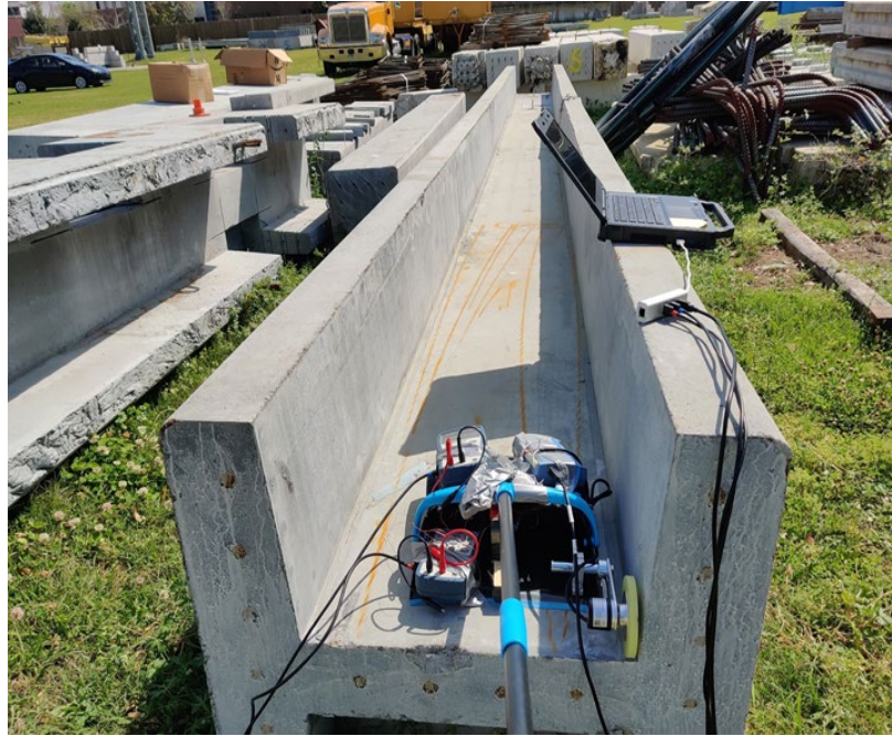
Figure 221: The field setup with the device on the H-pile
