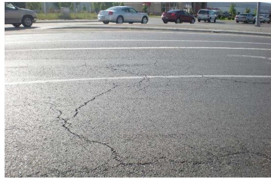
(b) Cracking
