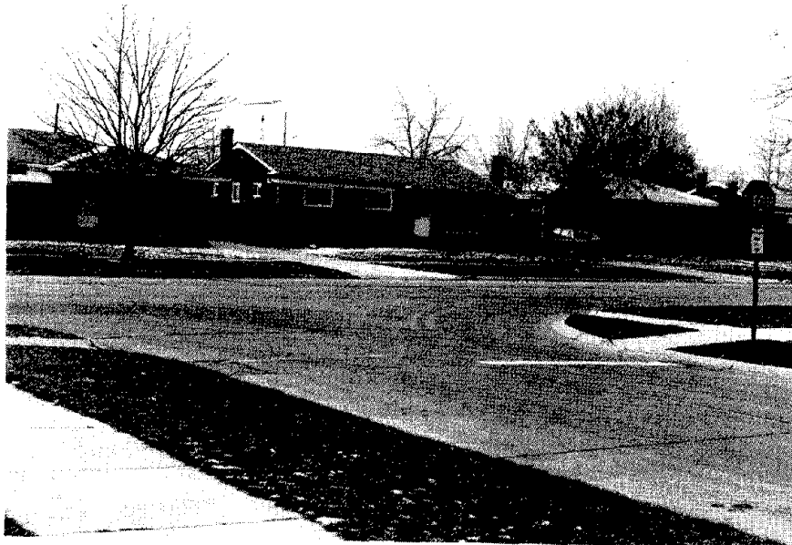
FIGURE 6. SUPPLEMENTARY SIGN AT T-INTERSECTION AFTER CONVERSION. (Text of sign as in Figure 5. Note use of stop line.) (TRENTON, MICHIGAN)
