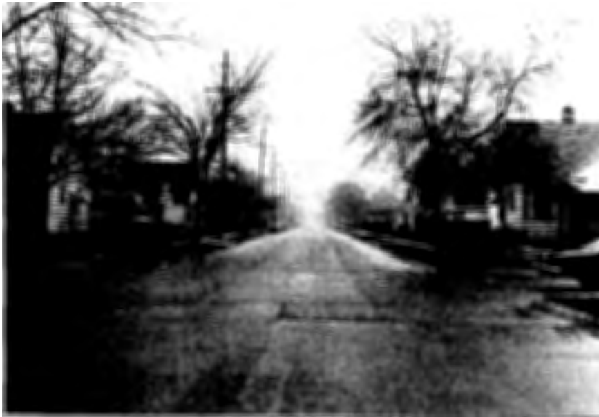
FIGURE 8. RESIDENTIAL COLLECTOR WHICH HAD 4 OF 16 INTERSECTIONS CONVERTED FROM 4-WAY TO 2-WAY STOP CONTROL. (BERKLEY, MICHIGAN)
