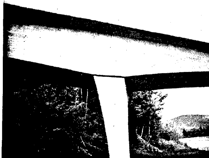
Figure 8. Closeup of bridge shown in figure 10 showing no signs of distress in spite of differential settlement of abutment.
