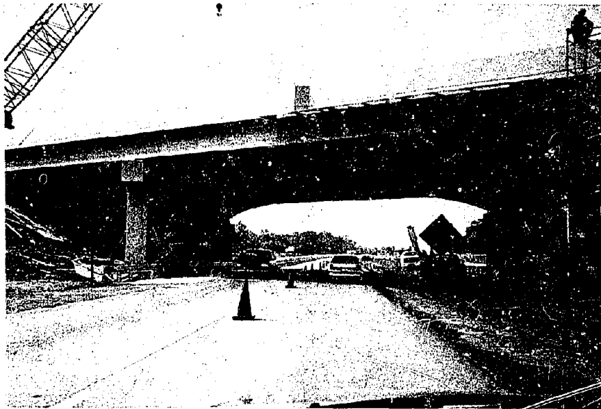
Figure 7. Temporary TLTWO with cones on I-75 in Kentucky.
