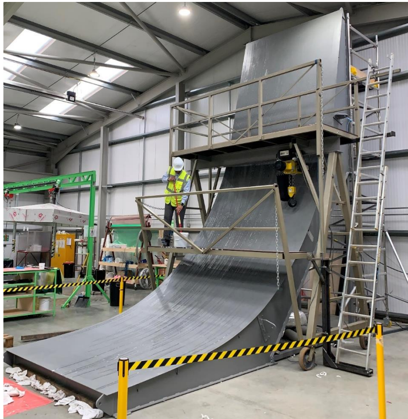
Figure 87: Gantry and scaffold tower installed around demonstrator tool
