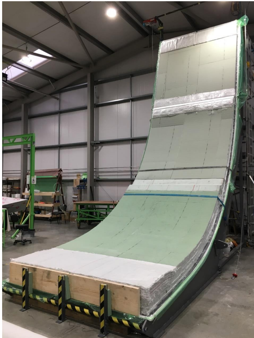
Figure 102: Outer skin and core layup completed
