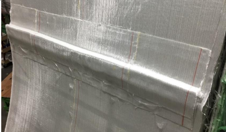
Figure 101: Joint 2 support layup. Photographs in order of production from top left to bottom right.
