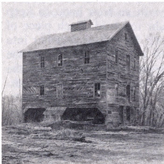
HILDEBRAND'S MILL FACING EAST
