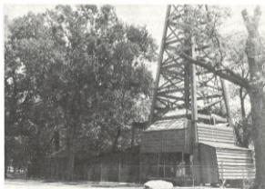
Redwood replica of the derrick with rigging on the original site of Nellie Johnstone No. 1, "Oklahoma's First Commercial Oil Well," in the Nellie Johnstone Park at Bartlesville.
