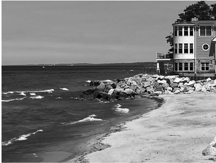
FIGURE 2. Image of property at the Michigan-Indiana border illustrating interruption to the ability to traverse a Great Lakes beach caused by the installation of hard armoring structures. (Credit: Photo taken by Norton, June 2022.)
