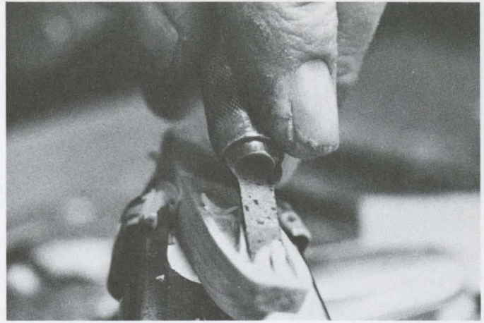
Gouging out the deck.
