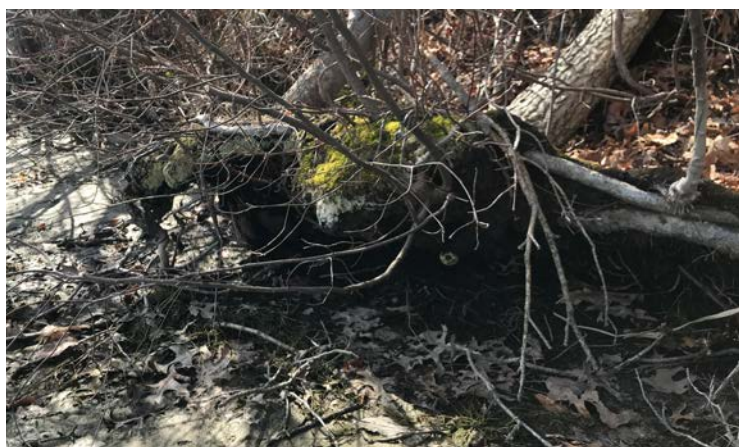
Fig. 4.5.2 The riverbank below the cemetery showing signs of erosion
