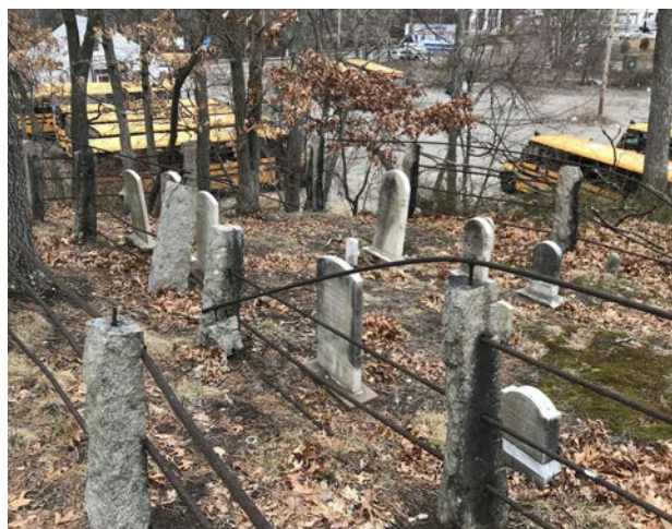
Fig. 4.5.11 The worst section of erosion, sloping away from the camera
