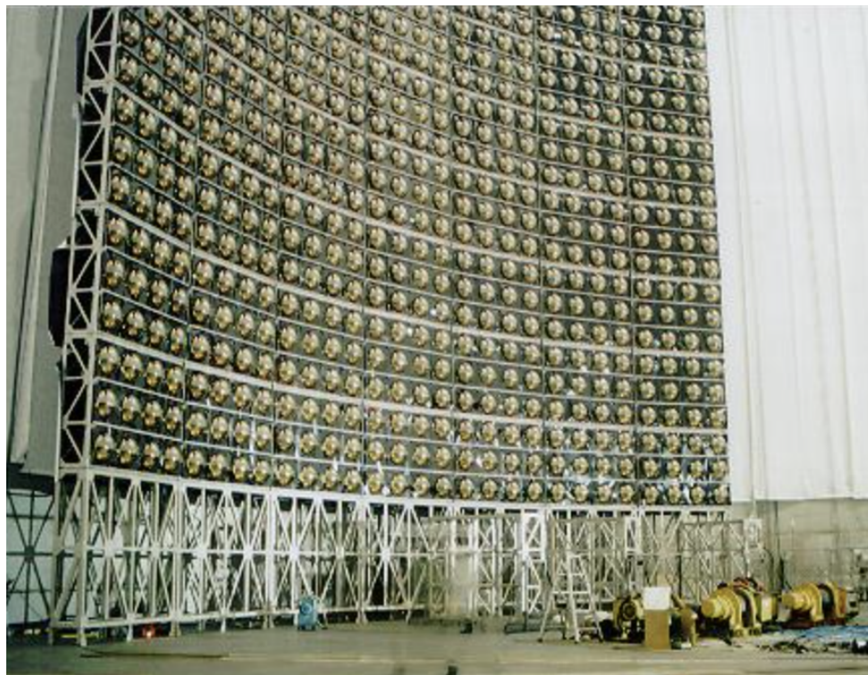
FIGURE 3.13: A PMT wall array during construction showing the Inner Detector (ID) PMTs around the tank wall. The steel framework structure holding ID PMTs can be seen. The Outer Detector (OD) PMTs are on the backside of the steel framework facing the tank wall. [85]
