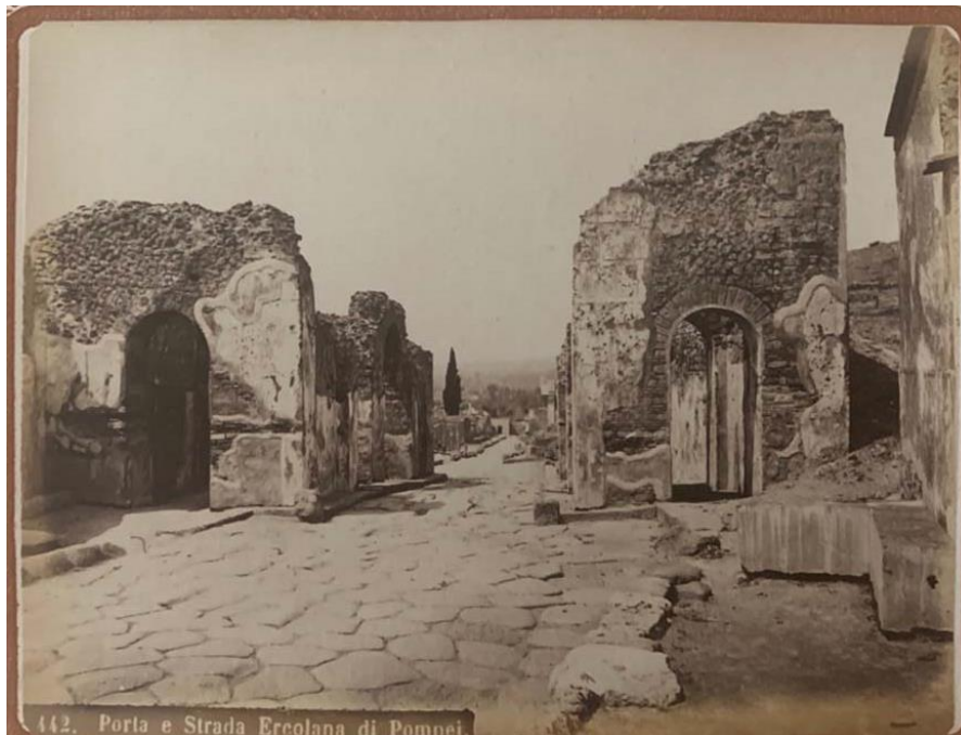
Figure 5.15 - View of the Porta Ercolano, dated 1868, showing additional plasterwork and damage to towers ( https://pompeiiinpictures.com/pompeiiinpictures/Gates/Gate%20Ercolano_files/image027.jpg ).
