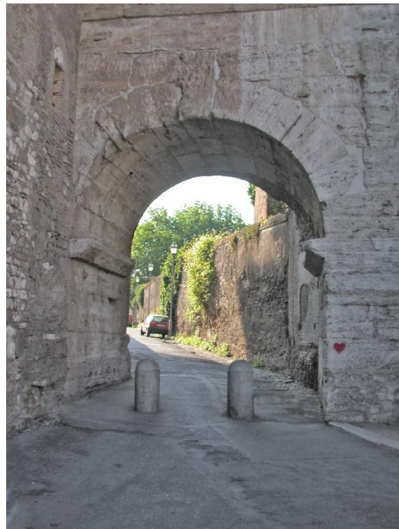
Figure 4.7 - Standing remains of the Porta Caelimontana, taken from the exterior of the gate. N.B. The modern height of the gateway is substantially reduced by later ground-level rise ( https://pt.wikipedia.org/wiki/Porta_Celimontana ).
