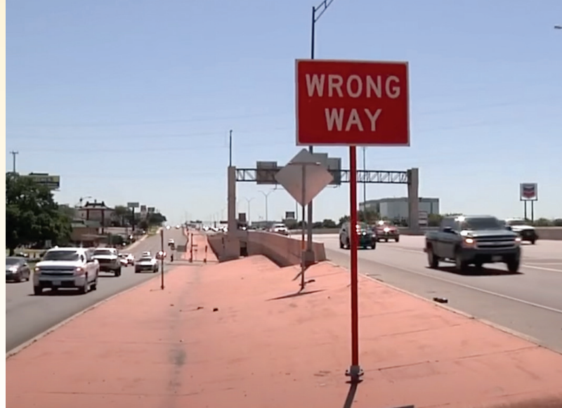
As a countermeasure, red reflective tape can be seen running down the entire length of the Wrong Way sign.
